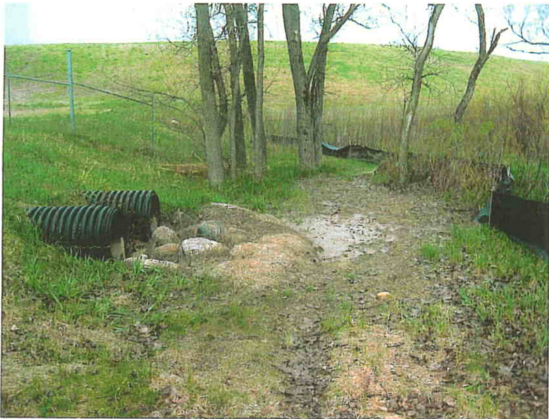
Figure 2-Place rip rap downstream of twin 30" culverts.
