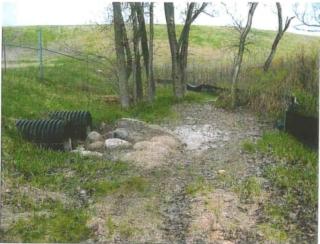
Figure 2-Place rip rap downstream of twin 30" culverts.
