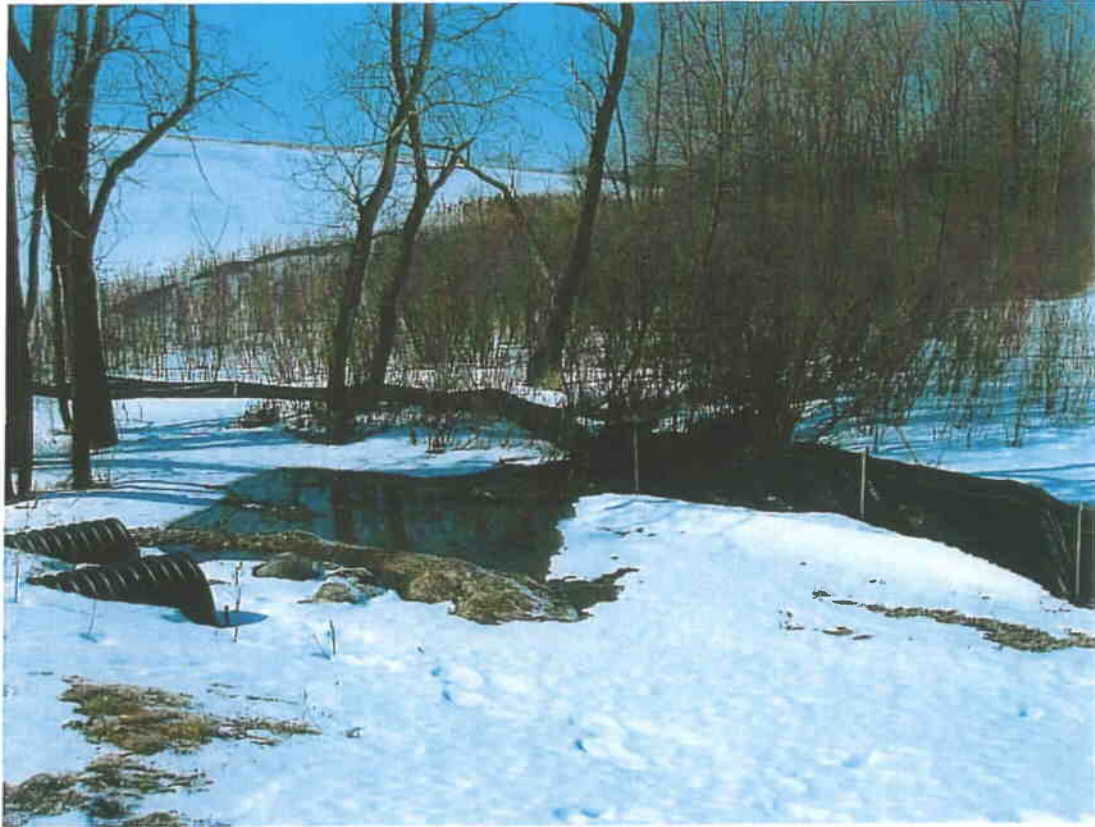
Downstream end of twin 30" culverts
