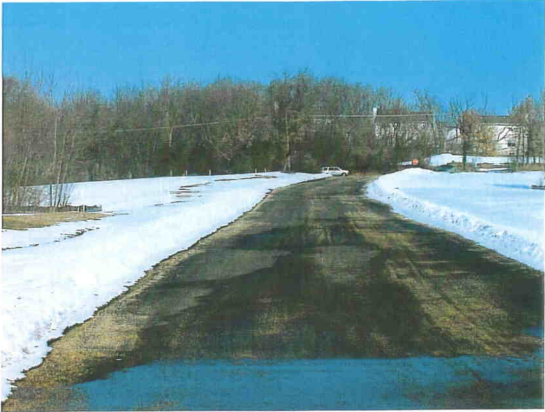
Entrance road looking north at Depot St.
