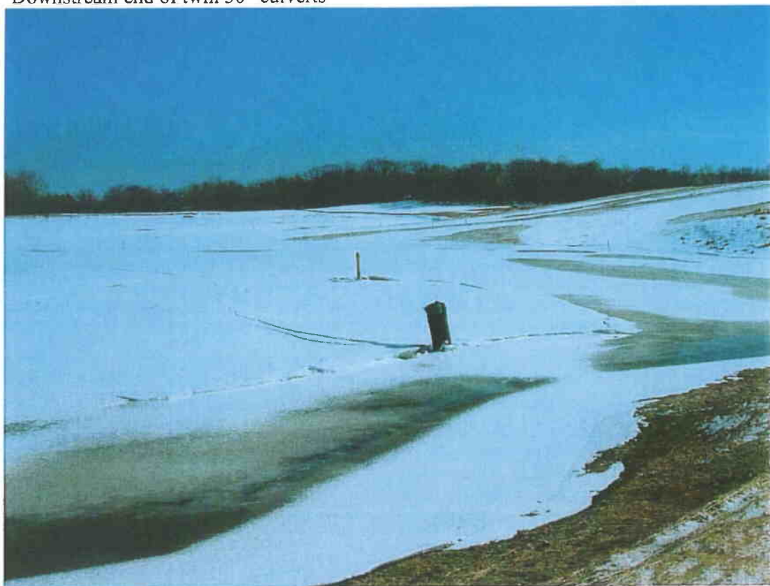
Temporary riser pipe
