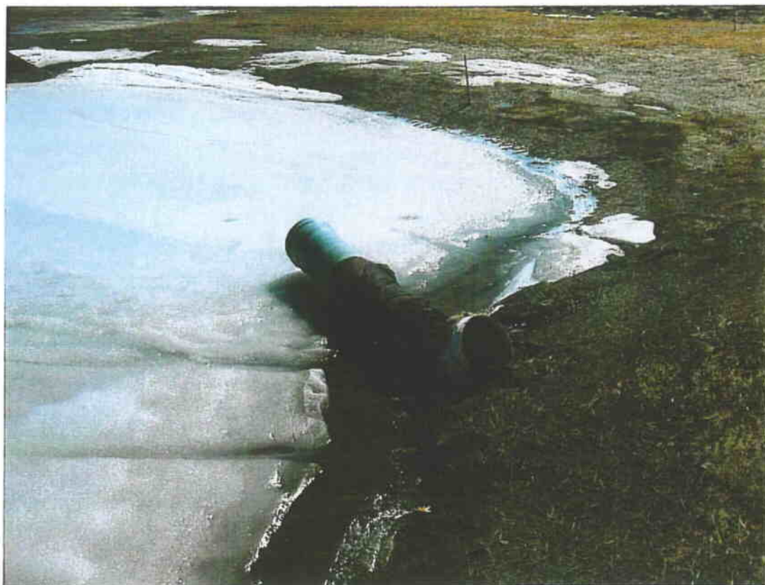
Figure 4-Re-set perforated riser in 12" flared end section SS#11.
