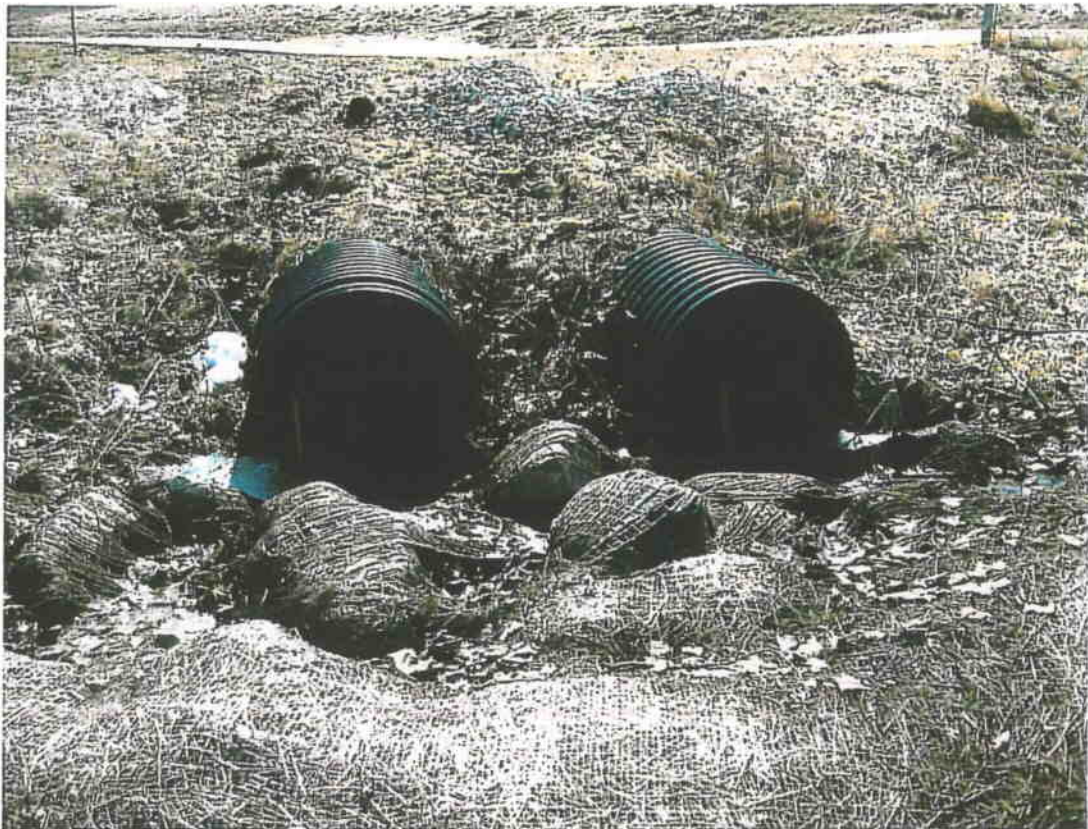
Figure 2-Install rip rap downstream of twin culverts.
