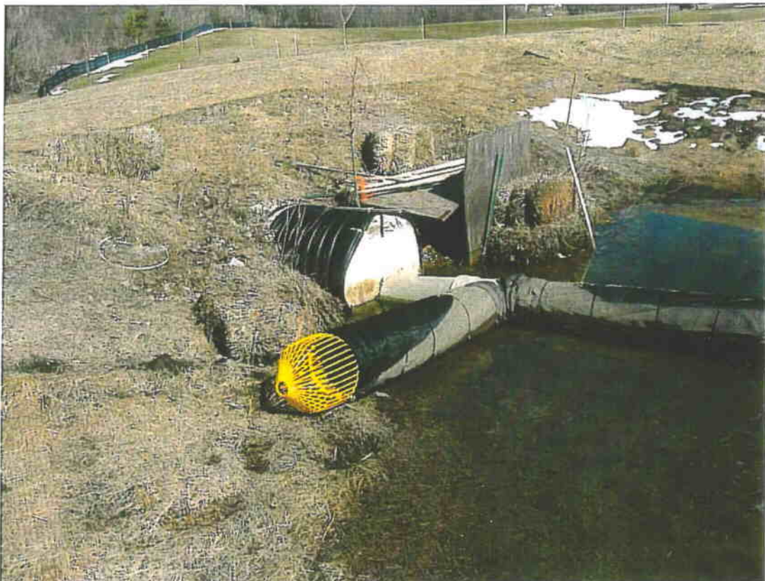
Figure 3-Re-set perforated riser to vertical position in 30" culvert.
