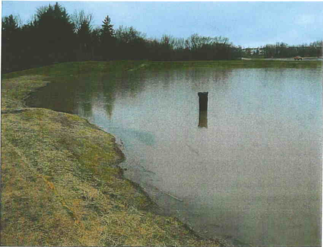
Figure 4-Perforated riser has been re-installed in pre treat area.
