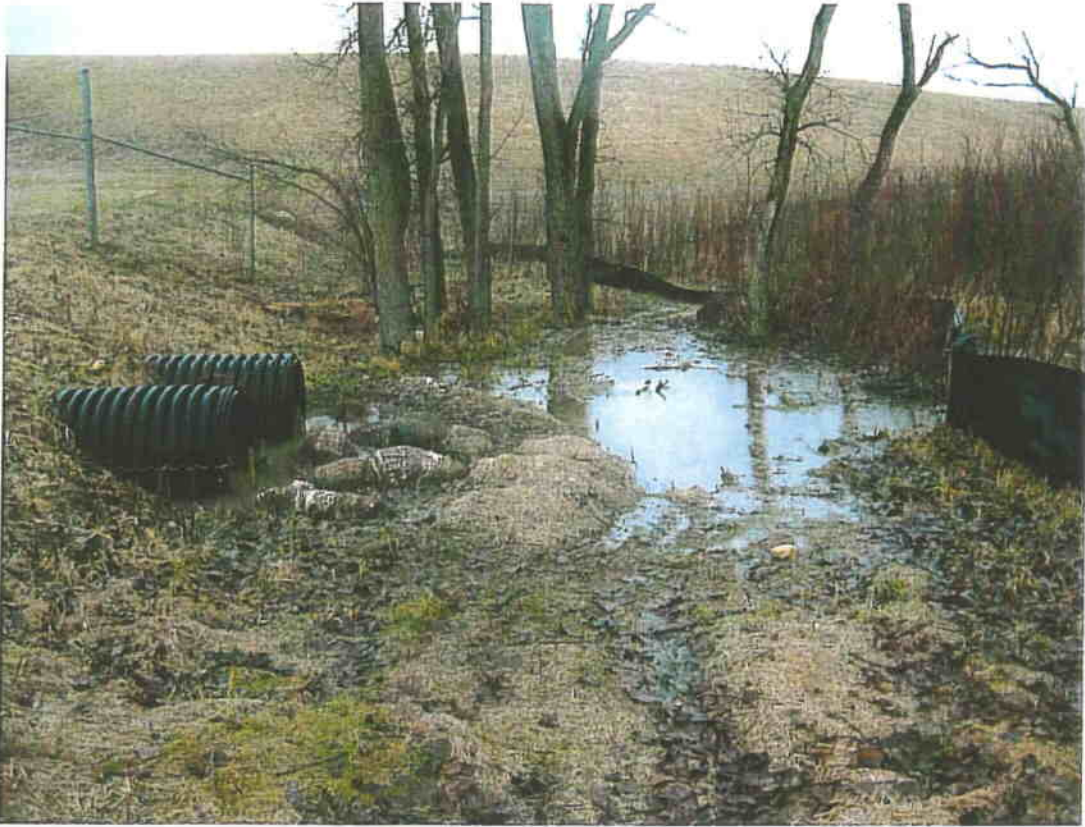
Figure 1-Install rip rap downstream of 30" culverts.
