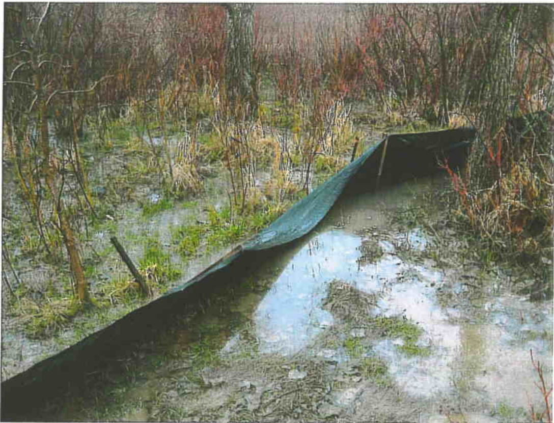
Figure 2-Repair silt fence downstream of 30" culverts.
